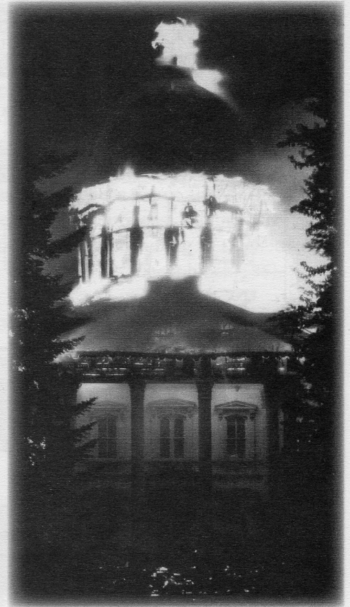
Capitol during the fire - courtesy of John Griffith
